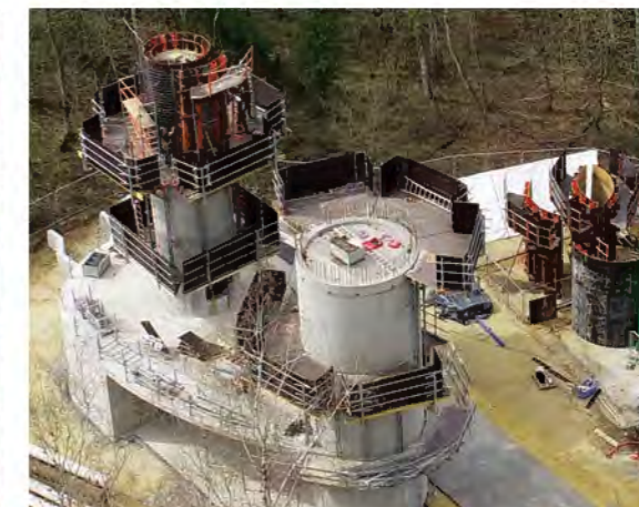
Construction des cuves © LSC-Group
