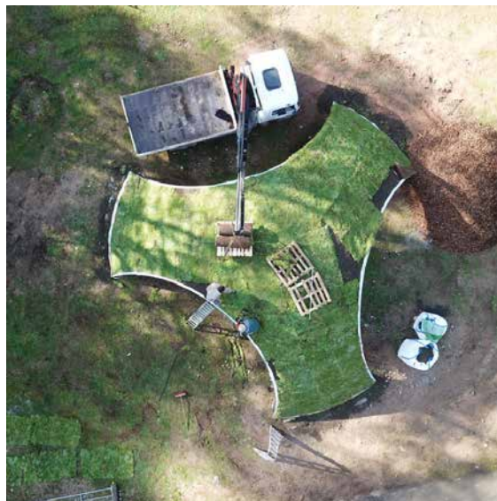
_DTC Recycleshell Demonstrator Green Roof Installation
