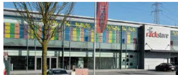
Retail Warehouse Foetz
