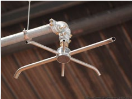
_Spray pattern realized by rotors
