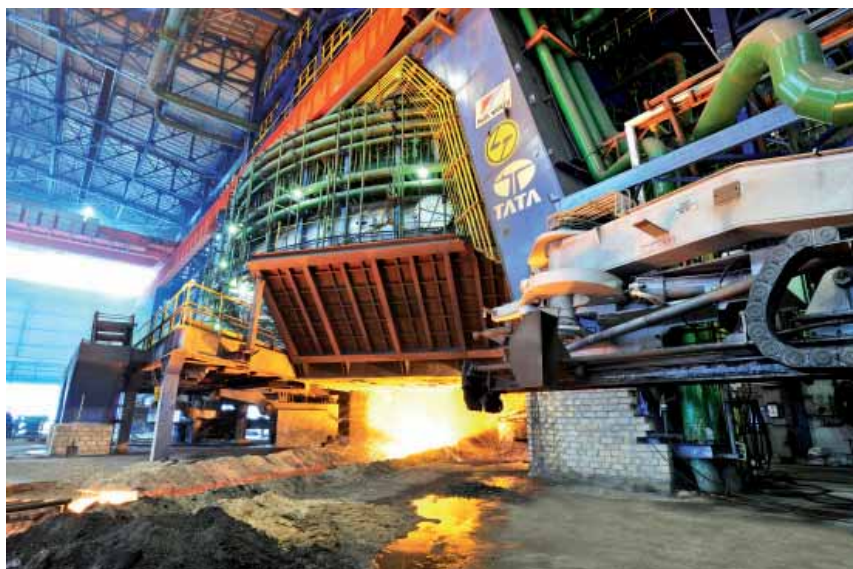
Tata Steel's Blast Furnace "H" at Jamshedpur, India – Casthouse
