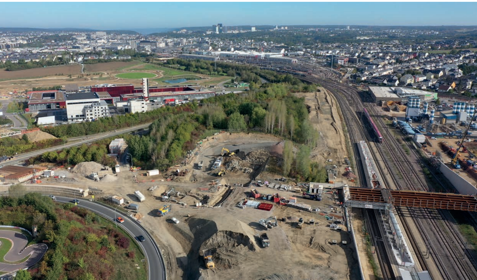
Chantier Gare routière Howald, Midfield © itchiban
